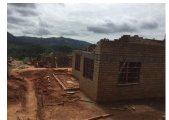
Nearly completed staff housing
