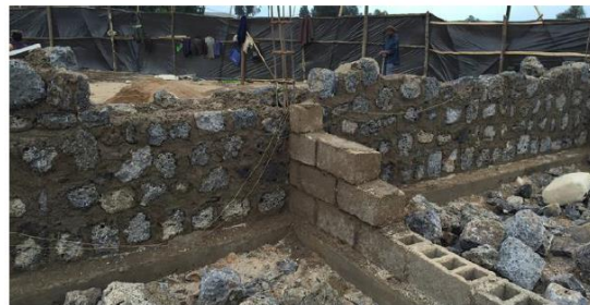
Elevations for the maternity block started.
