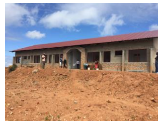
Completed Dambe Health Center
