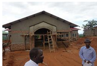
NSAMBE, MALAWI - FEBRUARY 10, 2015: Construction under way at the Dambe Health Center in Nsambe, Malawi. At left is APZU Executive Director Luckson W Dullie. (Photo by Todd McCormack / Partners In Health)
